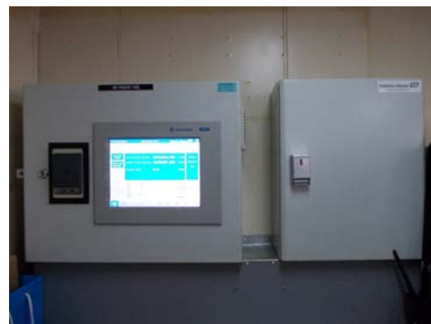
Wall mounting housing 600 x 400 x 210 mm and wall mounting control unit 400 x 500 x 210 mm
